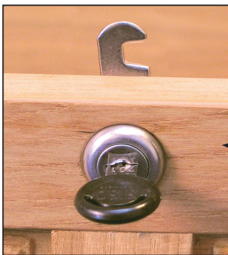
Close up of Cam lock
